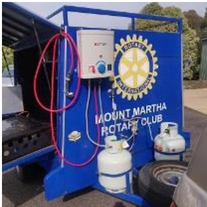
Operating mode showing Hot Water System
